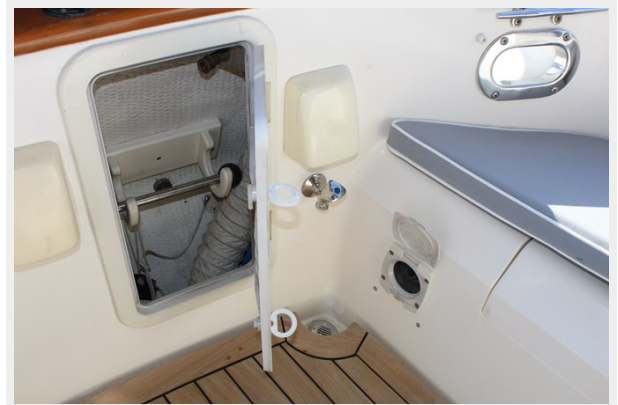
Emergency, manual bilge pump
