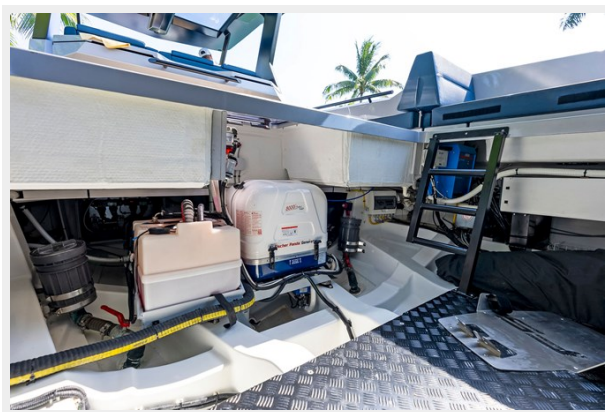
Storage, Housing Generator & Other Mechanics
