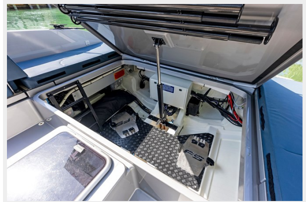
Storage, Housing Generator & Other Mechanics
