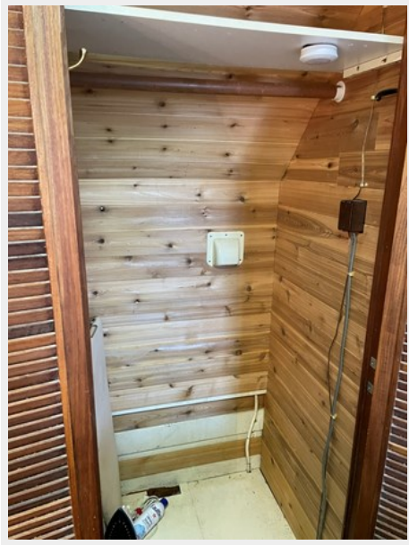
Aft center closet 1
