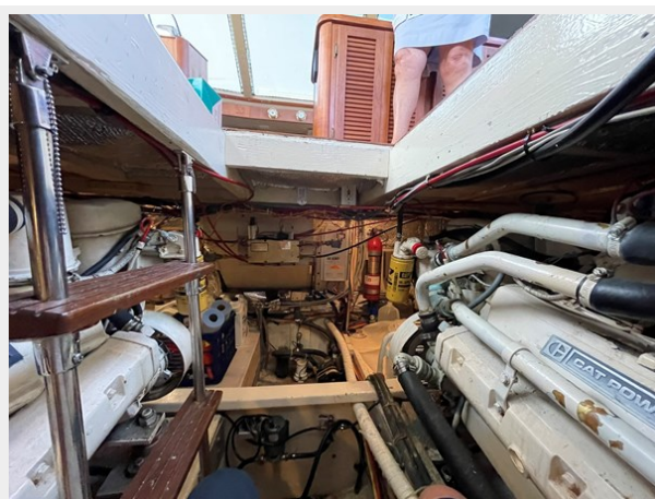
center line view
