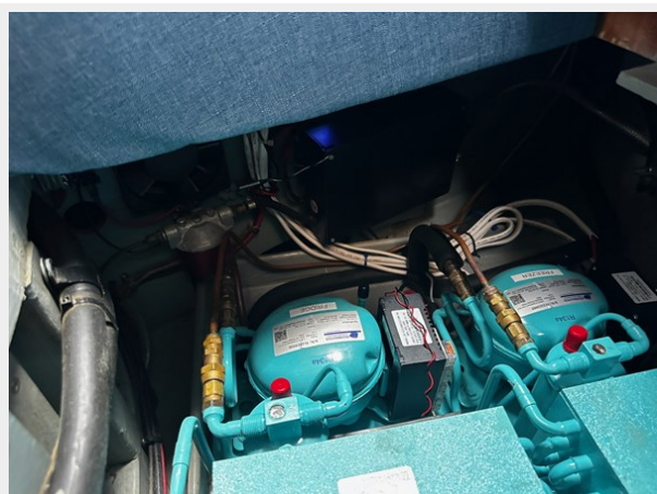
Refrig compressors
