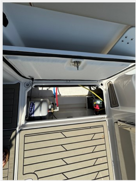
Hot Water Tank
