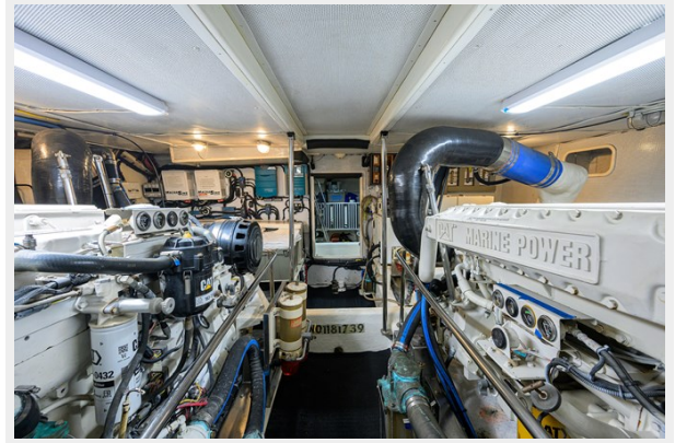
Engine Room Looking towards Lazarette
