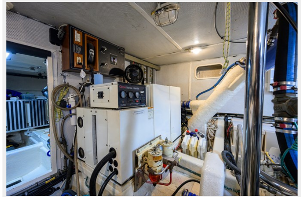
Engine Room Entry
