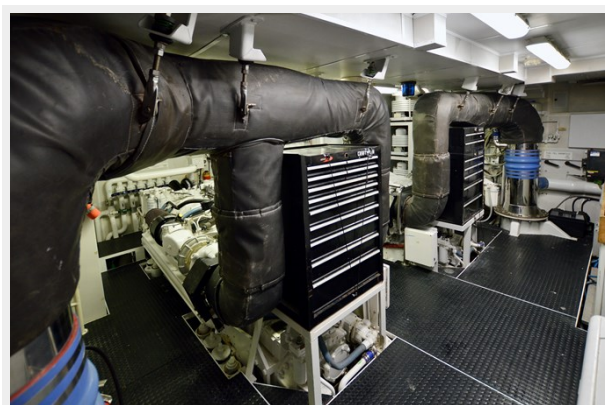
2001 DESTINY 98 ENGINE ROOM 2
