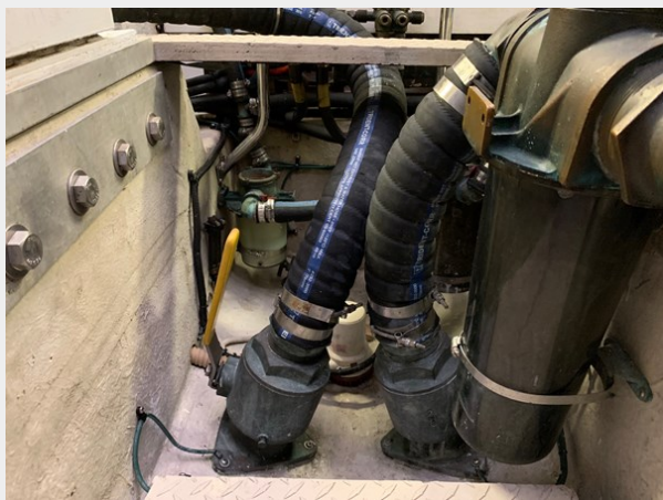
1995 SEA RAY 63 ENGINE ROOM 4
