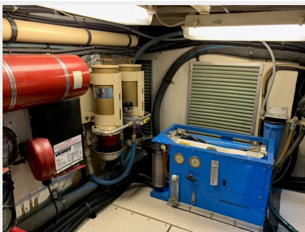
1995 SEA RAY 63 ENGINE ROOM EQUIPMENT
