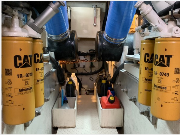
1995 SEA RAY 63 ENGINE ROOM 2
