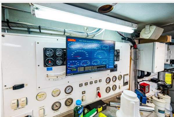
Engine Room Center
