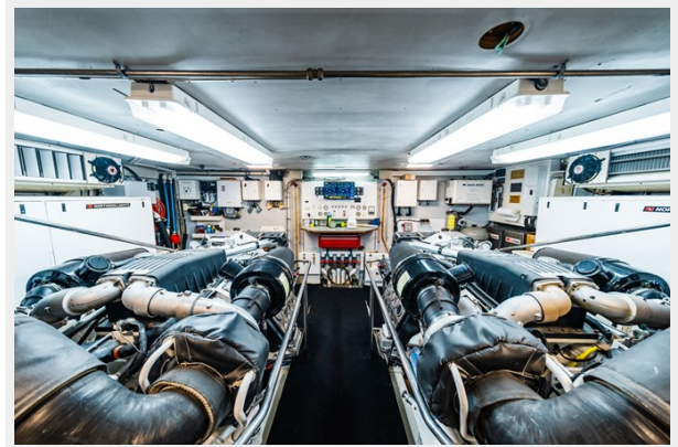
Engine Room Looking Forward
