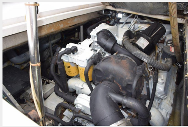
CAT 3208TA Starboard Side
