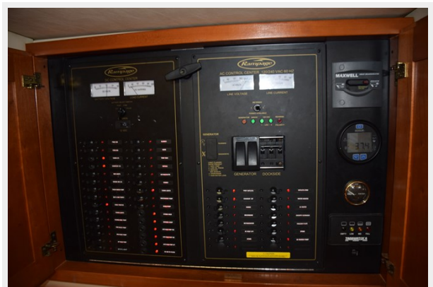
Primary Electrical Panel
