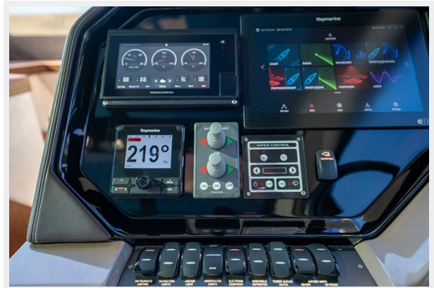
Main helm electronics/control panel
