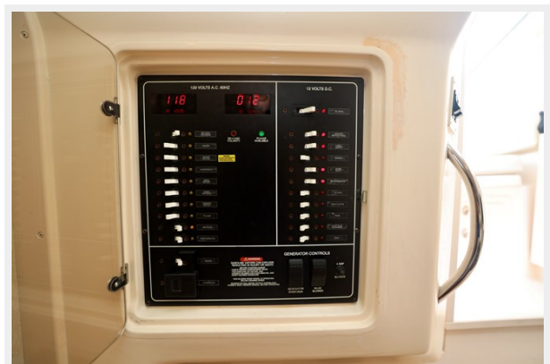
330 EXPRESS GRADY-WHITE 2003 ELECTRICAL PANEL
