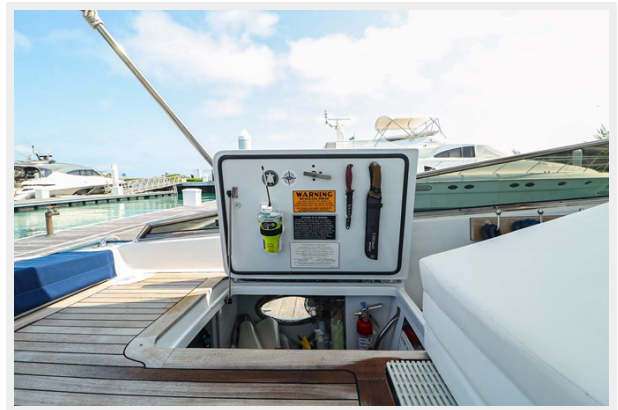
Access Hatch to Engine Room and Storage
