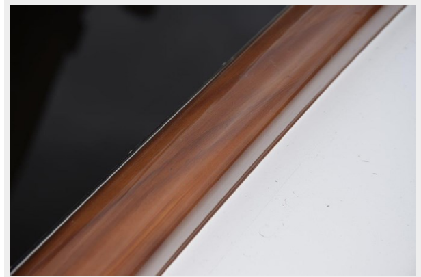
Faux finished toe railing
