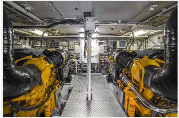
Engine Room Looking Forward
