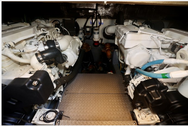
43 CARVER 2015 ENGINE ROOM
