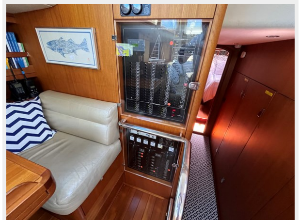
AC and DC distribution panel
