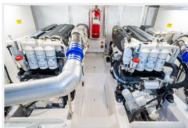
Maritimo M51 Engine room
