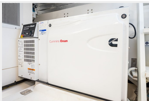
Maritimo M51 Engine room
