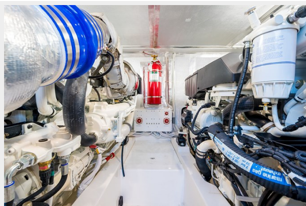
Maritimo M51 Engine room
