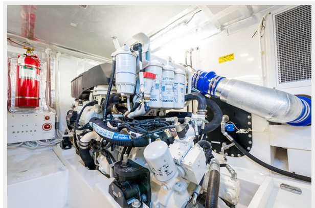
Maritimo M51 Engine room
