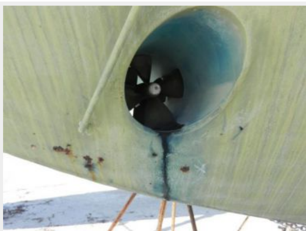
rust at concrete ballast at bow thruster
