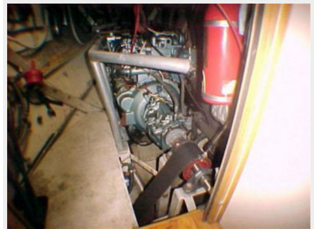
Engine room entry
