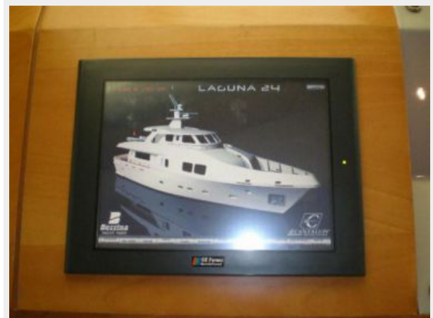
Systems monitor touch-screen control
