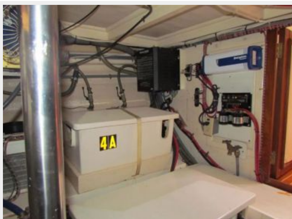
Engine Room Forward Port
