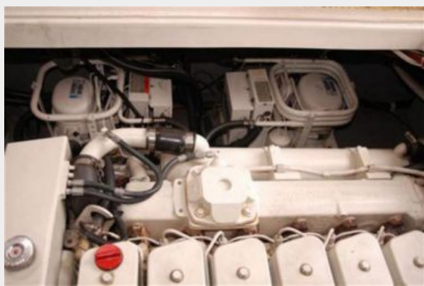
AC's Installed in Engine Room
