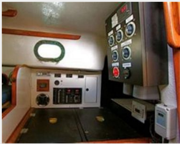
refrigerator and electrical
