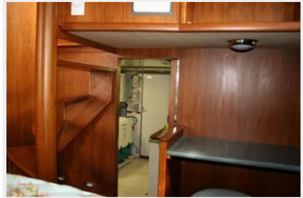
Access to Pump Room
